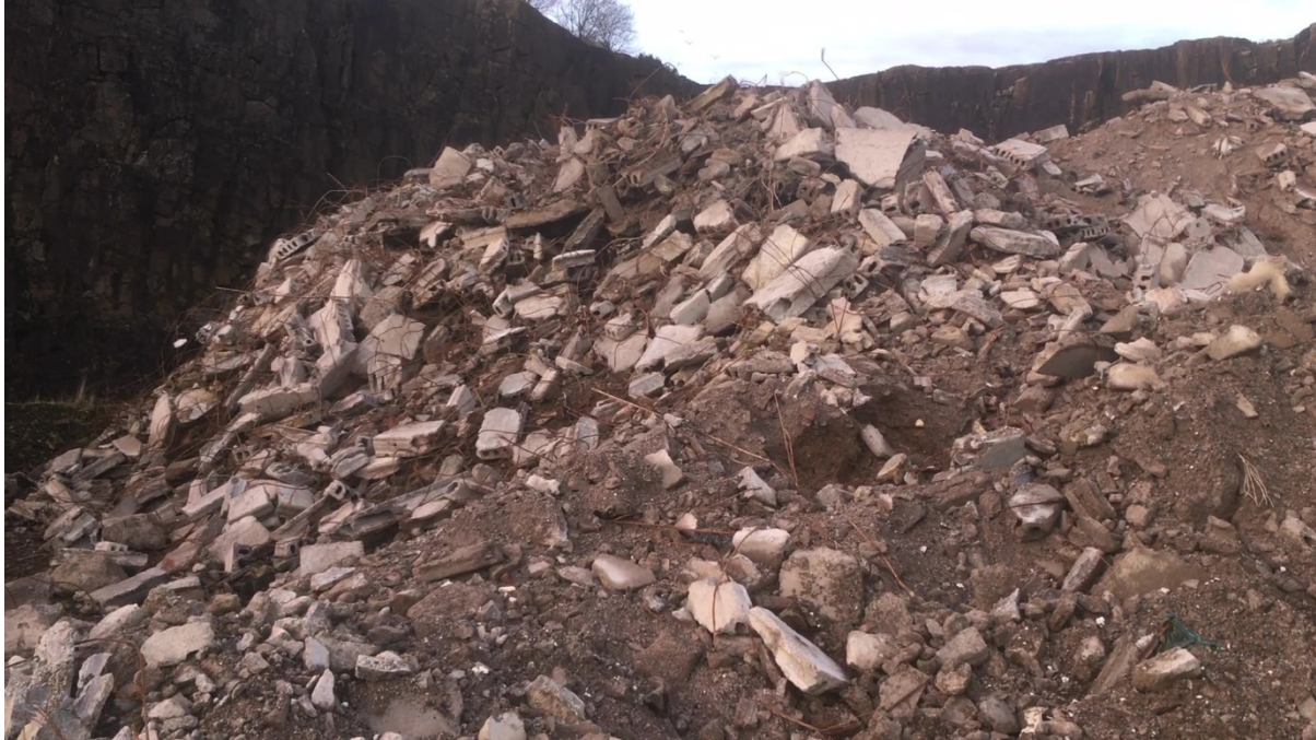
Above – Demolition material containing concrete and steel rebar, prior to steel removal
