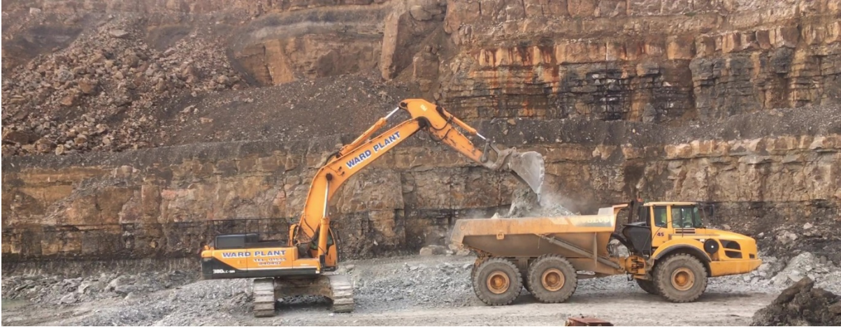
Above – Excavation area
