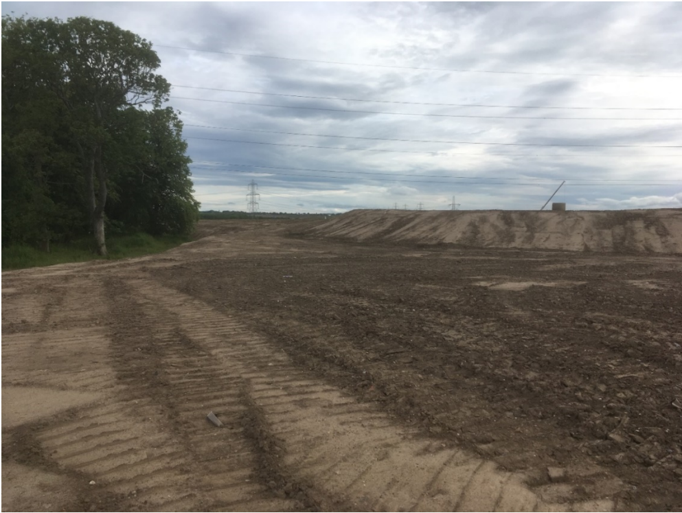
Advance - Newton Farm Phase 4 - 5 months
