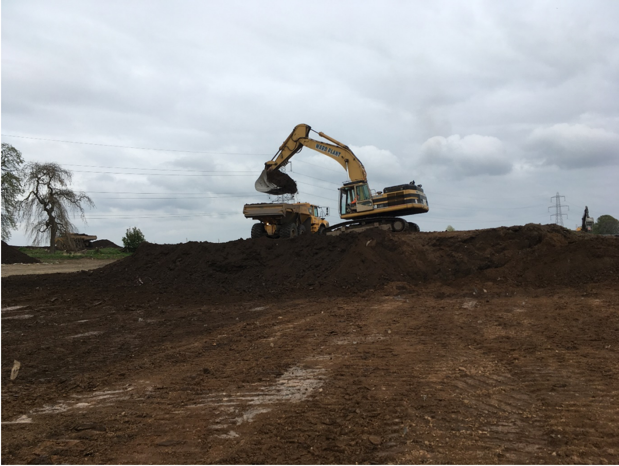
Advance - Newton Farm Phase 3 - 2 months
