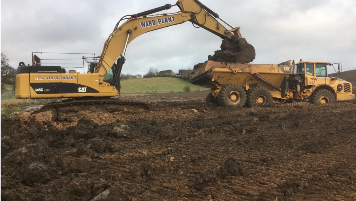
Advance – Newlands – ongoing
